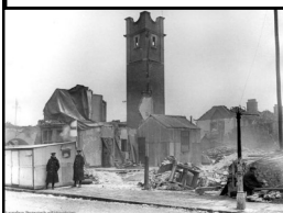
The destroyed Fire Station
