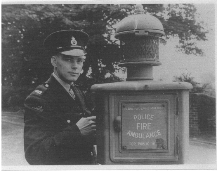
PC Eric Clark, Stone Division, Staffordshire Constabulary, at a Type PA1 pillar
